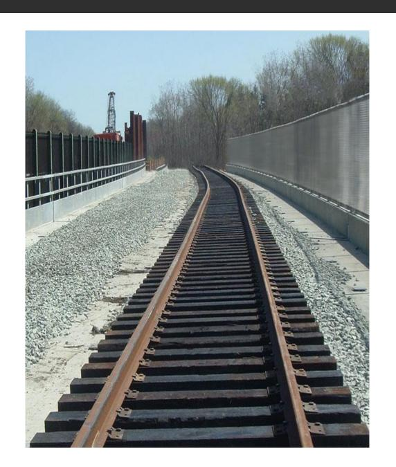
The wood physical and mechanical properties make it the ideal material to manufacture sleepers because it has the necessary strength and toughness to withstand heavy loads, but also has the flexibility that allows it to absorb vibration and "work" without crumbling or breaking.
